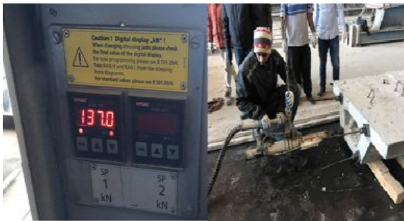
Fig. 4 Post-tensioning process of segmental beams and applying jacking force of 137 kN
