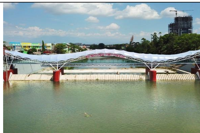
Fig. 2 Tirtonadi Weir in Surakarta, Indonesia
