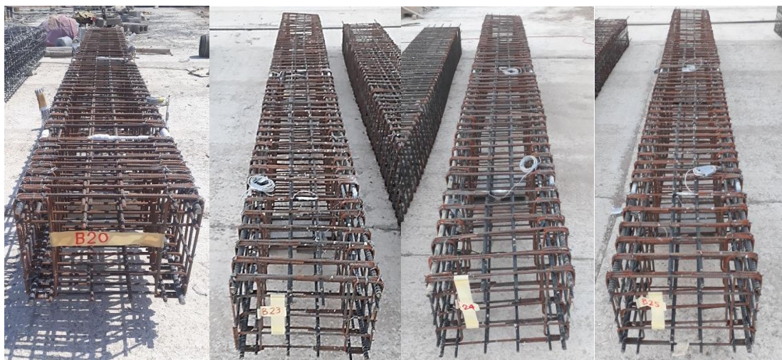
Fig. 2 Reinforcement cages
