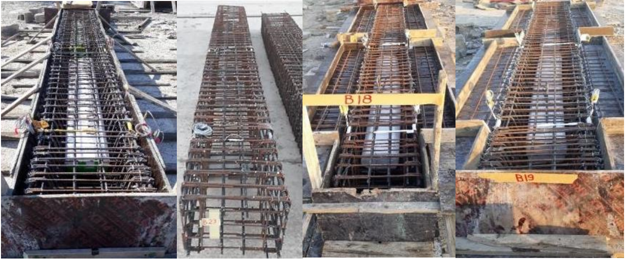
Fig. 2 Reinforcement cages and mold
