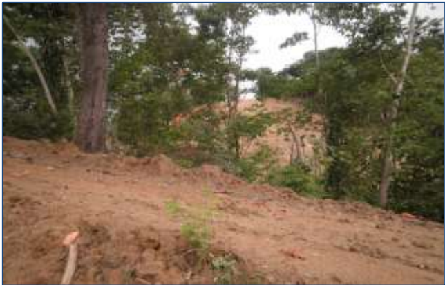
Figure 8. Land degradation due to soil erosion in Wai Samal Watershed
