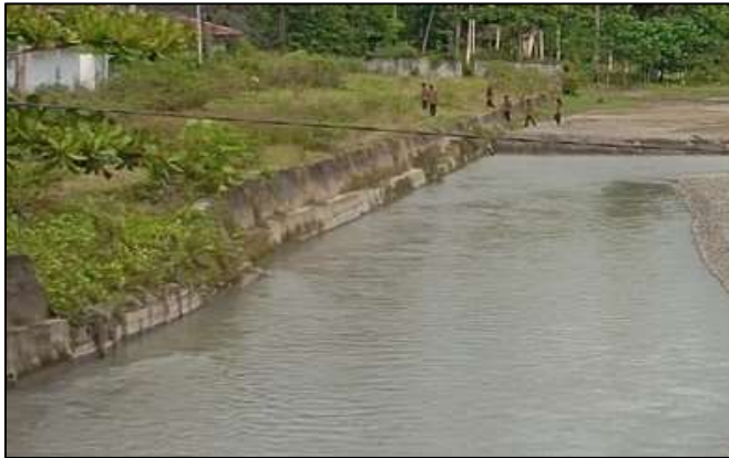
Figure 13. Sedimen load condition in the downstream of Wai Eti Watershed
