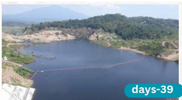
Fig. 4 Reservoir condition after initial filling (impoundment) on Day 39 (The authors)
