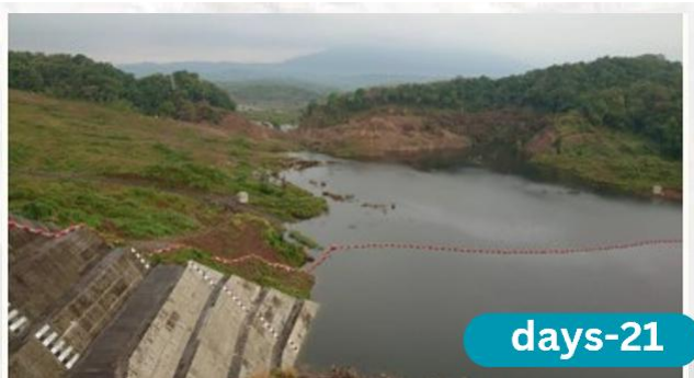
Fig. 3 Reservoir condition after initial filling (impoundment) on Day 21 (The authors)
