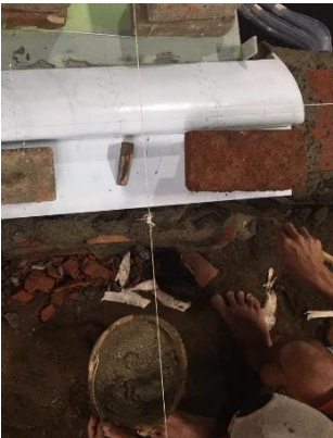
30 March 2021, placement of spillway merck
