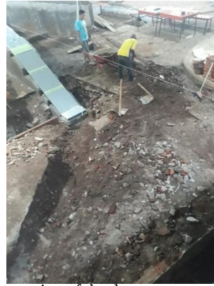
9 th April 2021, excavation of the downstream area for river contour
