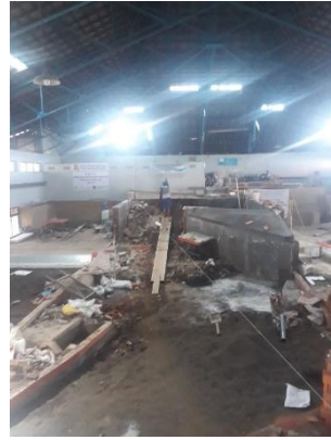
24 th March 2021, building stacking is almost complete
