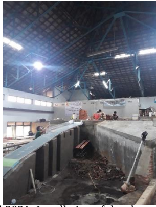
8 th April 2021, Installation of the chute way wall
