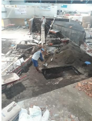
26 th March 2021, excavation on the location of the stilling basin
