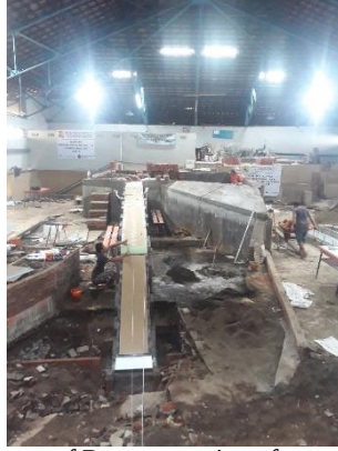
7 th April 2021, placement of R at connection of approach channels I-II and II-III
