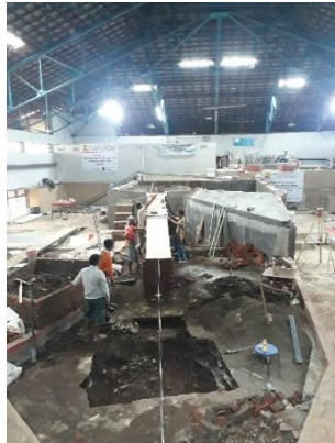
1 st April 2021, placement of approach channel II
