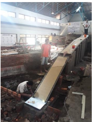
5 th April, 2021, placement of approach channel III
