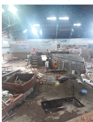
29 th March 2021, placement of approach channel I
