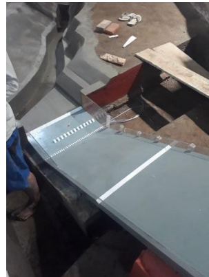
23 rd April 2021, Installation of barrier block at stilling basin
