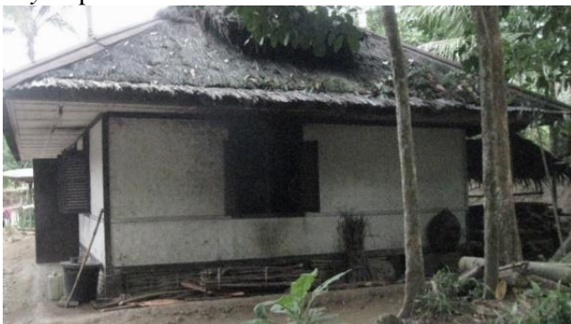
Fig. 3 Stilt house with kiray roof and cubicle walls
