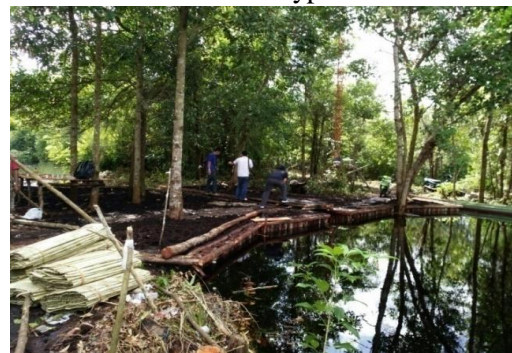
Fig. 8 Canal-blocking structure of semi-permanent using the local wood of Tumih tree type
