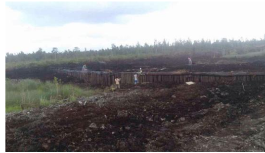
Fig. 12 Canal-blocking structure of semi-permanent using the local wood of the coconut tree with the width of the channel cross section of 50 m
