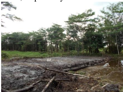
Fig. 10 Canal-blocking structure of semi-permanent using the local wood of the coconut tree with the width of the channel cross section of 25 m
