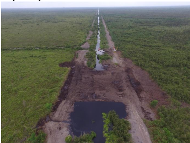
Fig. 6 Canal-blocking structure of compacted peat dam
