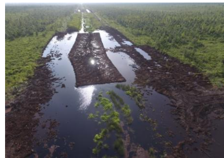
Fig. 4 Canal-blocking structure of back filling
