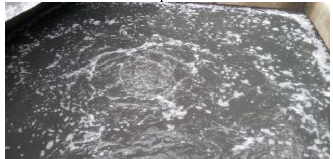
Fig. 17 Homogenization tank after Fenton application
