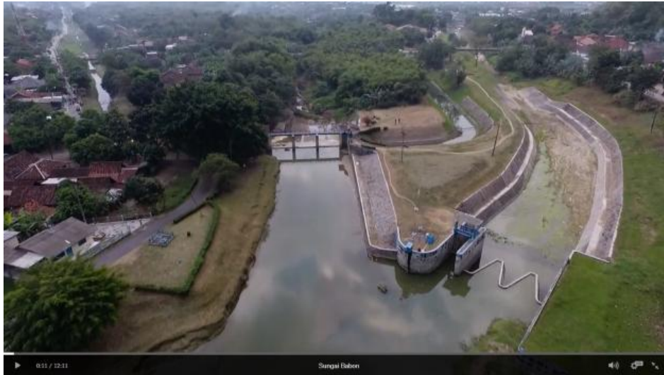
Fig. 3 Photos at Pucang Gading Weir on the Babon River
