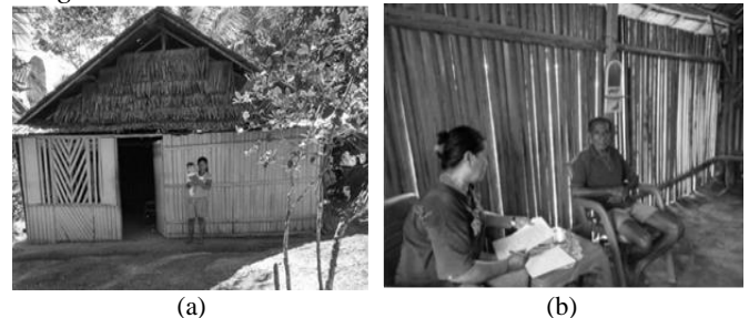
Fig. 2 a) The condition of one of the houses in the Land of Lumoli whose roof and walls are derived from a sago tree; b) House wall made of sago branch (gaba-gaba) split is arranged simply, traditionally, and not neatly to be easily penetrated by wind and cold air from outside, and the floor is ground
