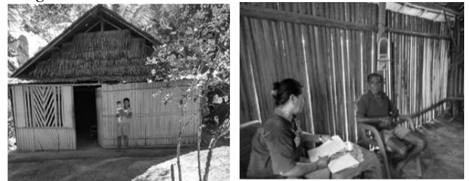
Fig. 2 a) The condition of one of the houses in the Land of Lumoli whose roof and walls are derived from a sago tree; b) House wall made of sago branch (gaba-gaba) split is arranged simply, traditionally, and not neatly to be easily penetrated by wind and cold air from outside, and the floor is ground
